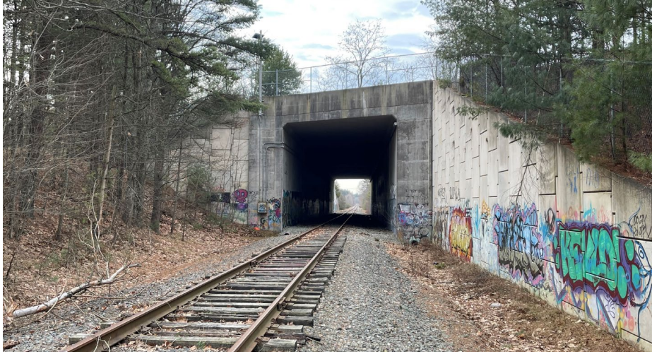
Route 196 – Topsham (Single Track Bridge)
