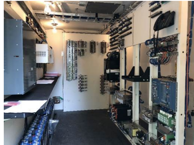
Signal Bungalow Interior
