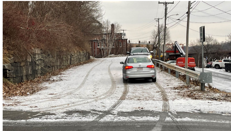
Bridge Street / Parking Area – Augusta (Tracks Removed)
