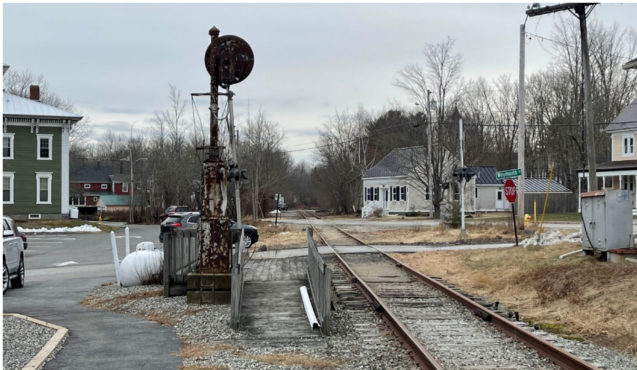
Weymouth Road – Richmond (Former Platform & Signal)
